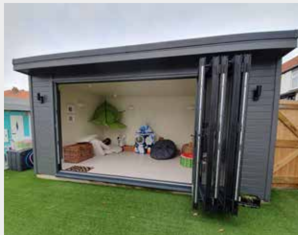
16' X 10' Pent garden studio, thermowood cladding, Aluminium 5 leaf 12ft bifold doors, painted finish in charcoal, MDF (V grooved) painted lining (white) with breathable membrane (moisture barrier) and Celotex insulation, painted finish in charcoal, EPDM rubber roof, laminate installed by customer & black guttering
